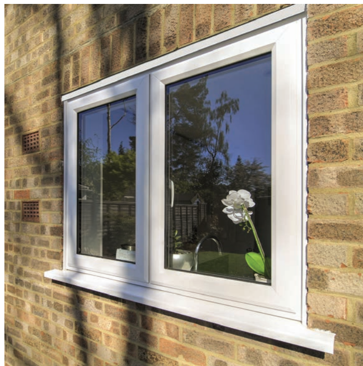
Concealed Ventilation installed through the outer frame
