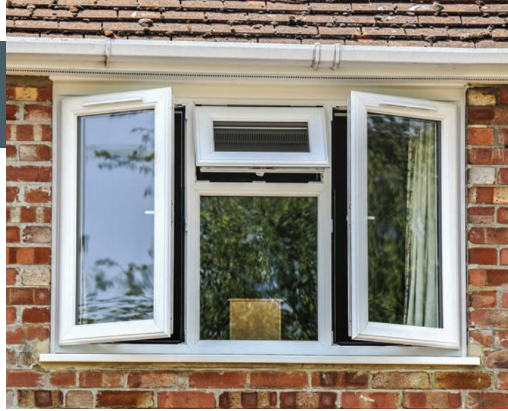
Trickle Vents installed through the window sashes
