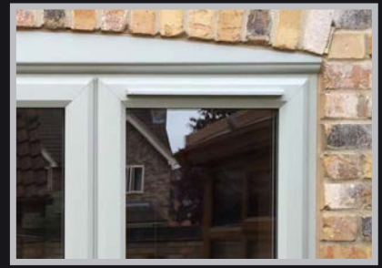
Trickle vent through a Rebated Sash
